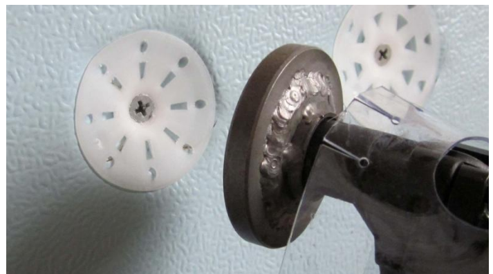
Plasti-Grip® CBW & CBW2 on Thermax® ci
