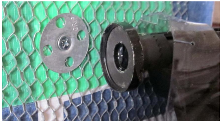
1¼" dia. Grip-Plate® on Metal Lath
